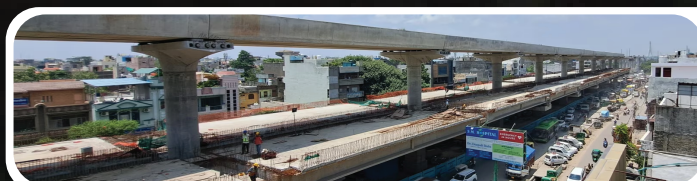
Railway, Metro & Bridge Projects
