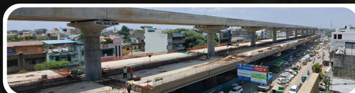
Railway, Metro & Bridge Projects
